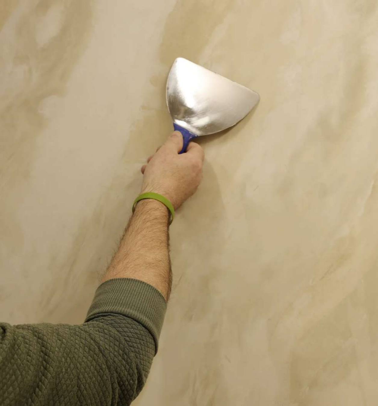
Application of Decorative Finishes
